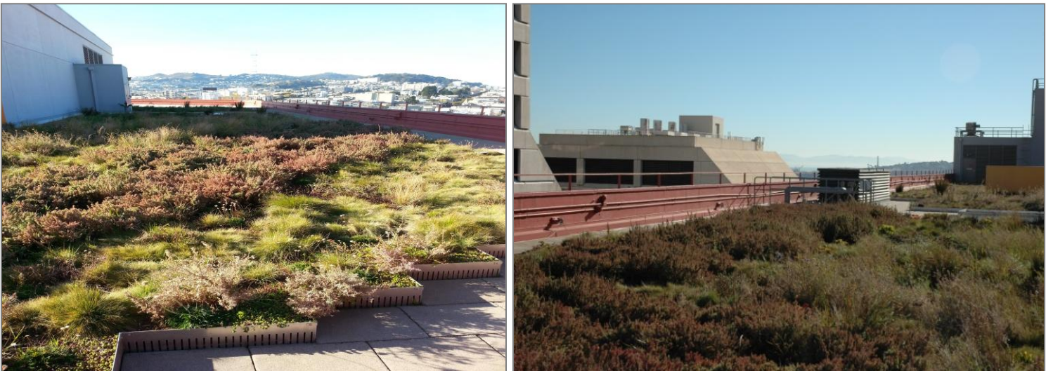
One South Van Ness Green Roof
