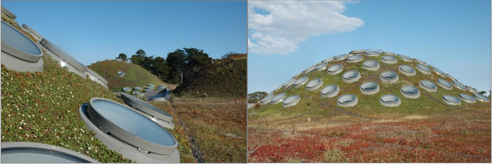
California Academy of Sciences Green Roof
