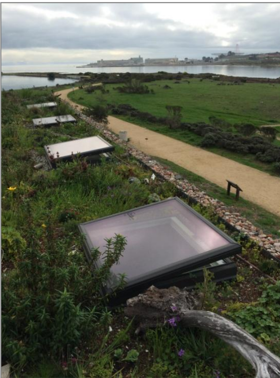
EcoCenter Green Roof (1)
